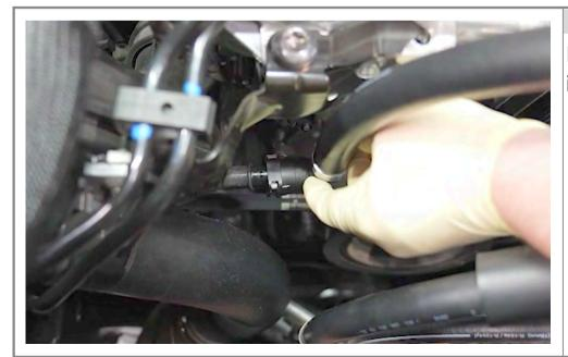
Step 25 pt.2 Install the 90° end to the intake pipe.
